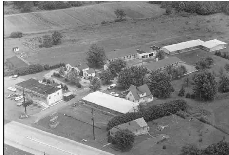
This aerial view was taken around 1961 and shows the motel when there were 33 rooms and the diner.
