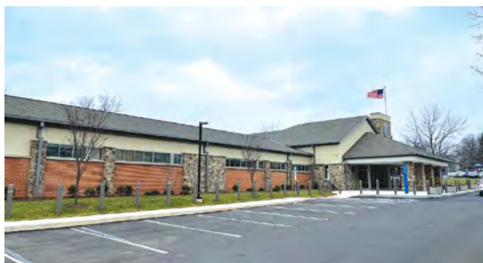
New Police Facility
