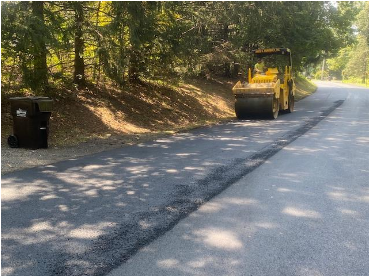
2021 Road Paving – Upper State Rd.
