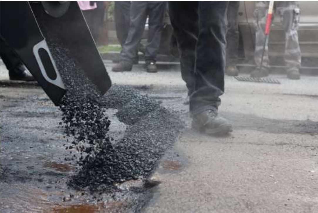
Parking Lot Paving
