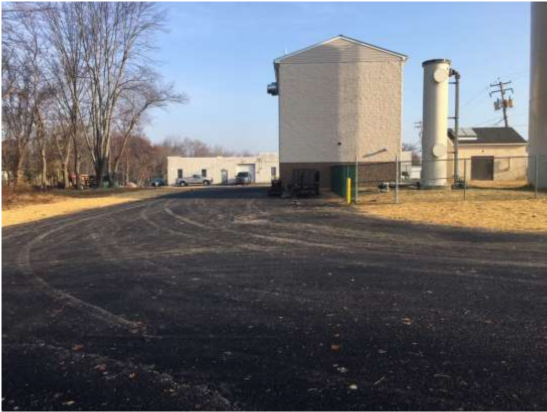
Costner Filtration Building
