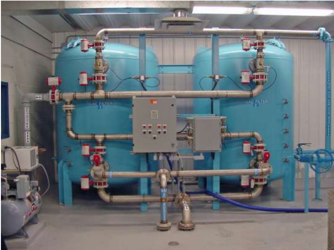
Granulated Activated Charcoal System
