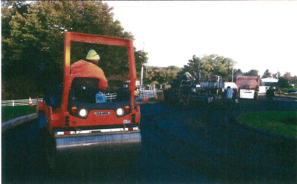
Township Building Parking Lot gets a much needed facelift!
