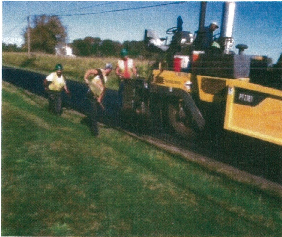
New Paving on Pickertown Rd.
