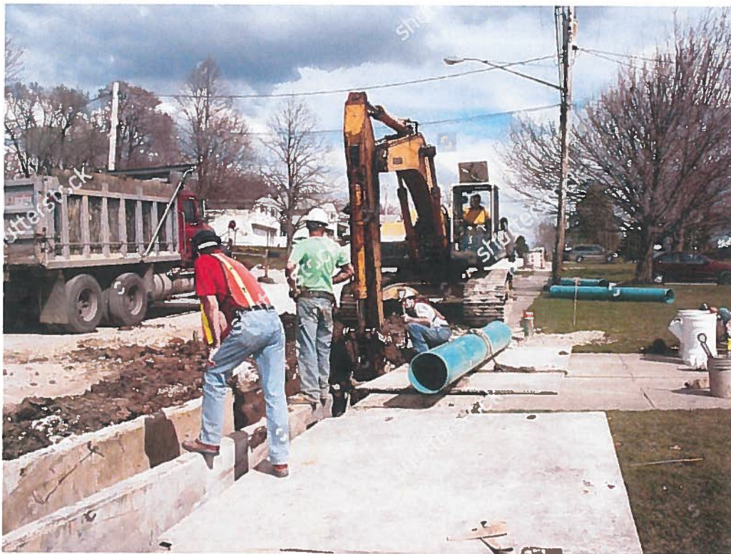
Installation of Sewer Lines
