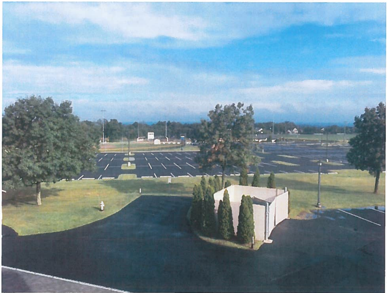
Expanded Parking Lot at Barness Park
