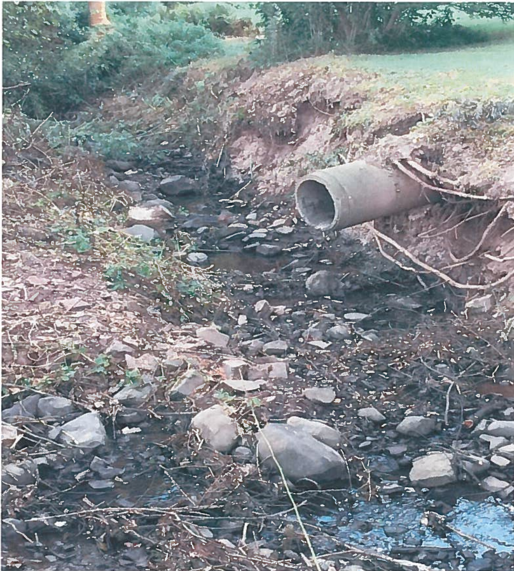
Palomino Streambank Stabilization Project
