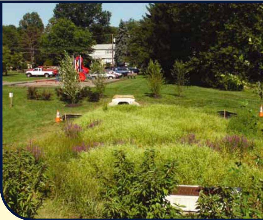
This man-made basin can hold a lot of extra water during a rainstorm
