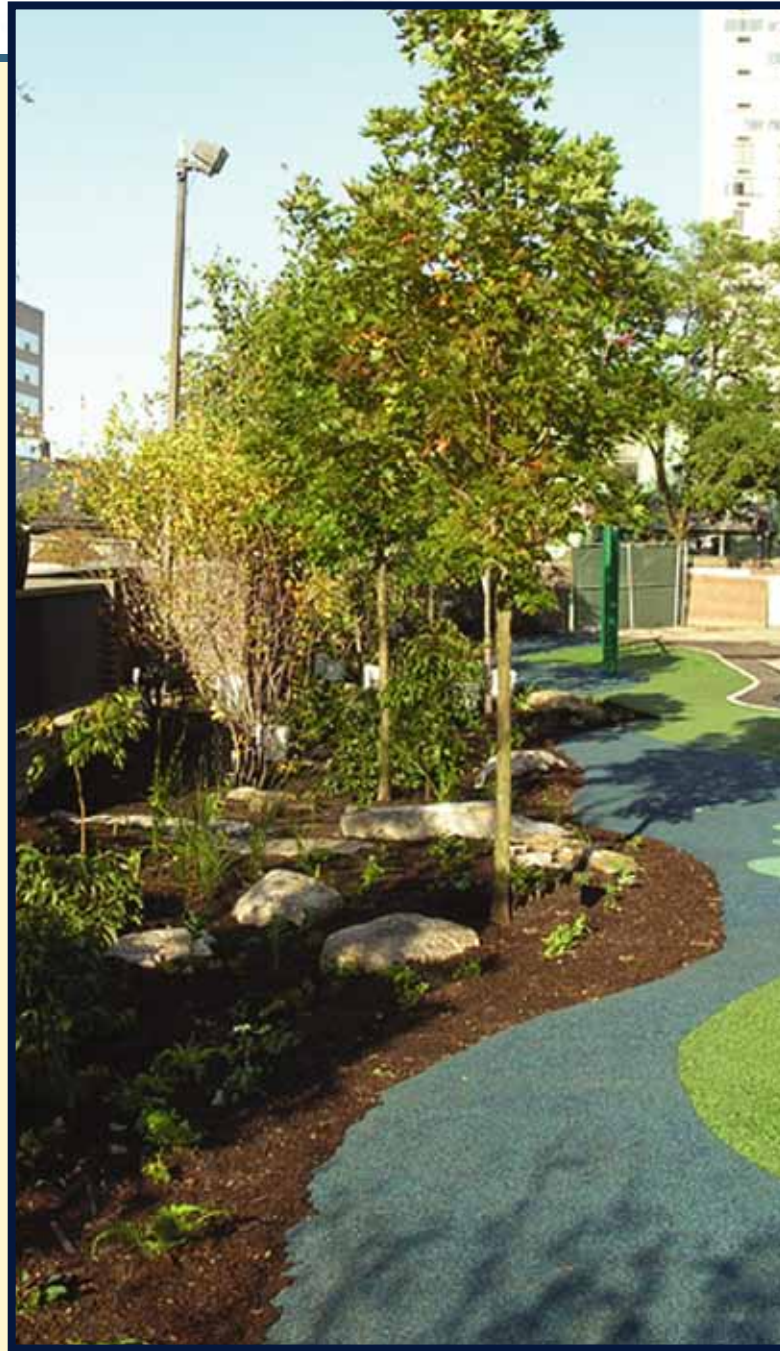
A rain garden alongside a porous play surface at Albert M Greenfield School
