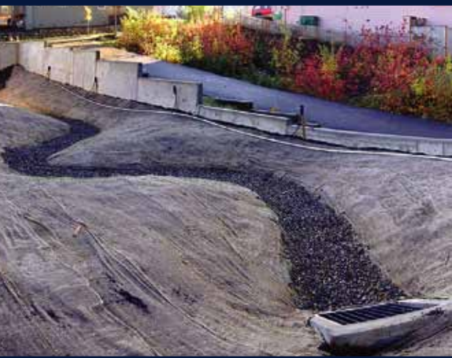
Meandering swale under construction
