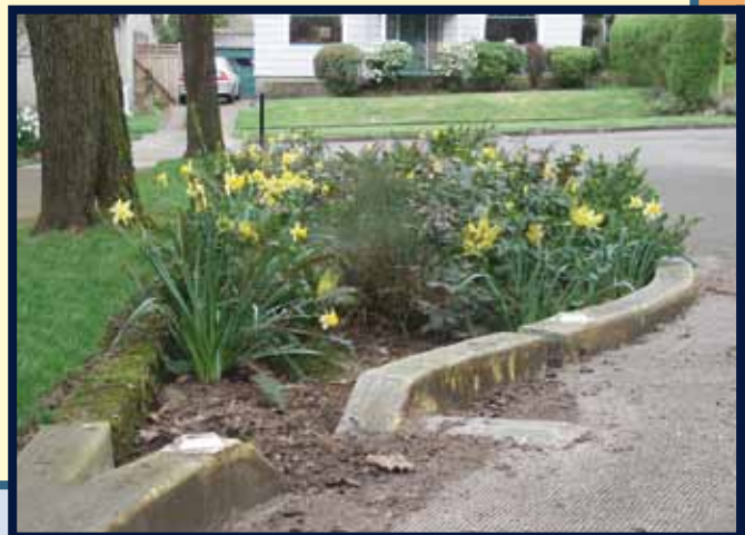
Stormwater curb bumpout in the neighborhood of Siskiyou, Portland, OR
