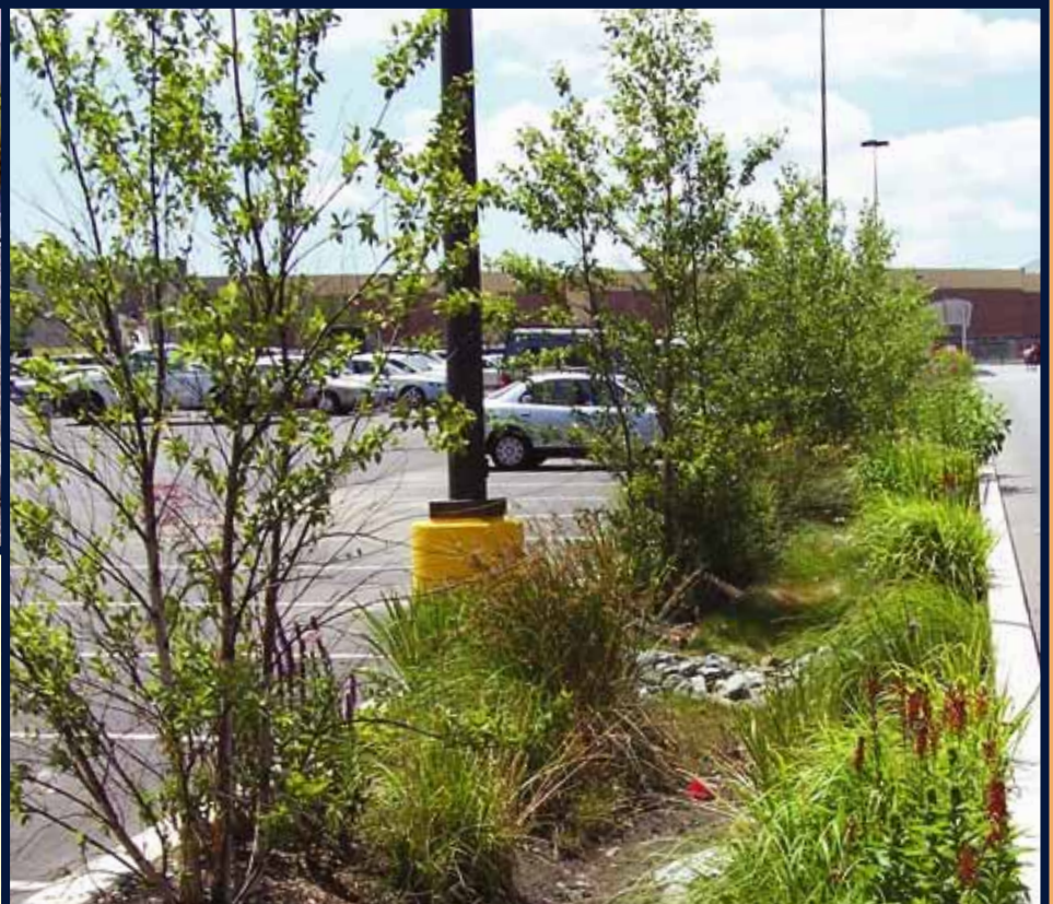
Recently planted vegetated swale in a parking lot
